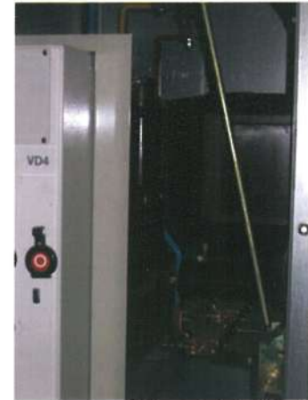
Earthing Switch Installation
