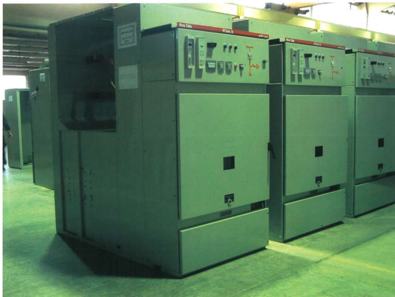
36 KV, 1250A ,25KA/3s NT-SAFE36 Type Tested withdrawable design
